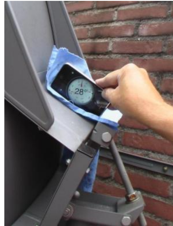
Elevation is the up/down angle that the dish is pointed
